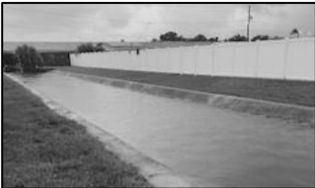
The culvert behind the villas on Larchmont Place
