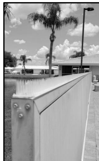
Defender Spikes Installed
