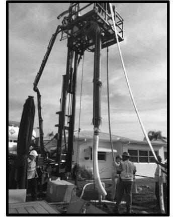
Sewer relining work in progress behind units on Heatherglen Drive
