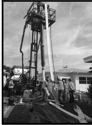
Sewer relining work in progress behind units on Heatherglen Drive
